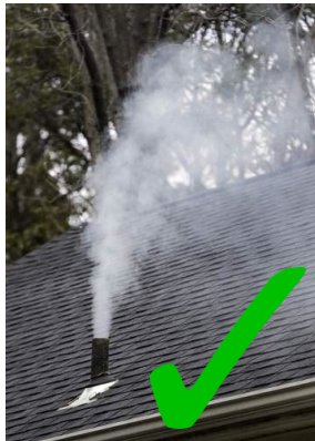
Smoke from roof vent OK
